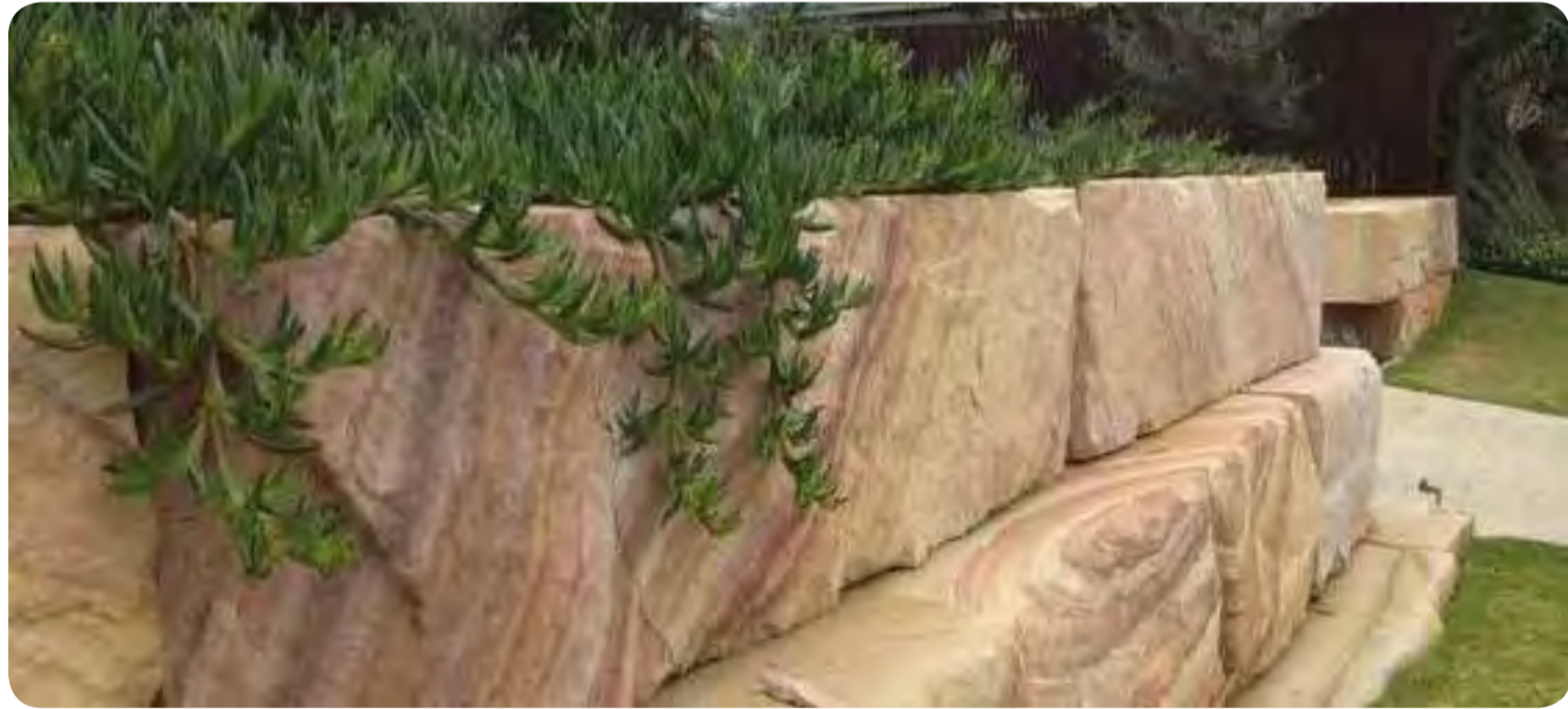
Sandstone block retaining walls
